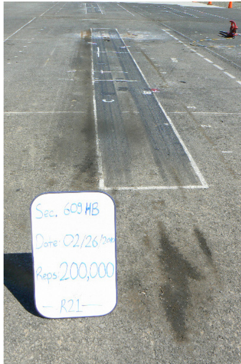
Figure A.13 609HB - PG 64-28 PM - 114 mm: Section photograph at test completion.
